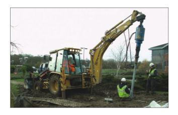
The conventional foundations are uneconomical and consumes enormous time. Hyquip through its intensive study and trails has come up with different types of foundations like Screw pile, Precast surface mounted and Under reamed precast structures to suit various soil conditions and to ensure speedy installations.
